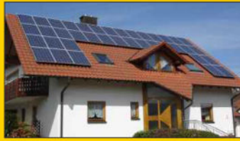
Off-grid home solar system
