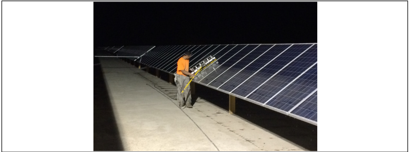
Picture 3: Clean the modules in dark or when it is cool outside. This reduces evaporation of water.
