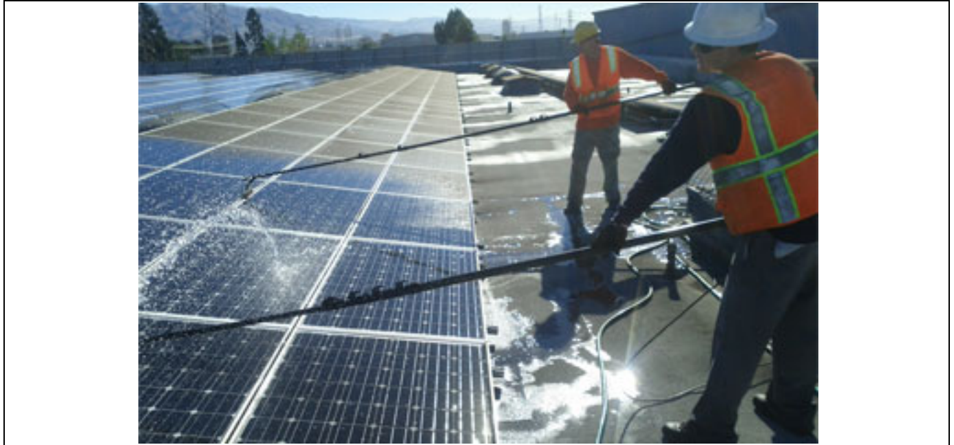
Picture 4: Typical cleaning process with water and squeegee
