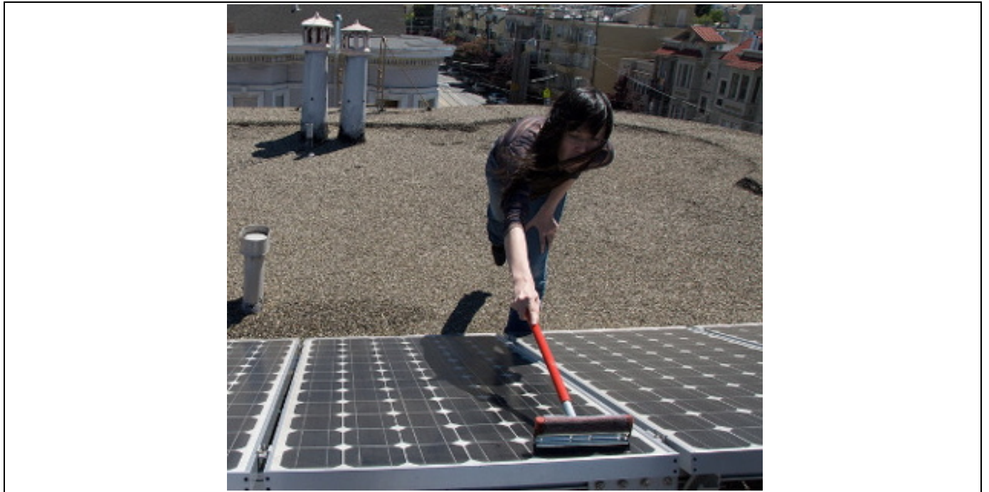
Picture 2: Proper grounding of cleaning personal and cleaning direction
